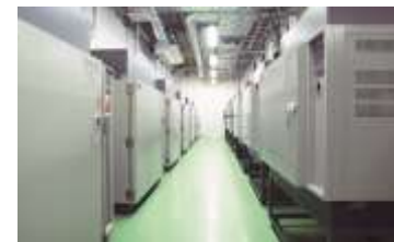
■ Thermostat inspection chamber
